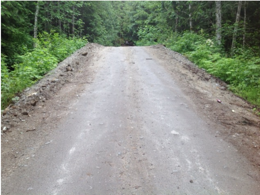
Approach from Right Bank when facing downstream
