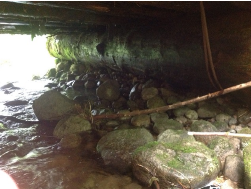
Right Bank Abutment when facing downstream
