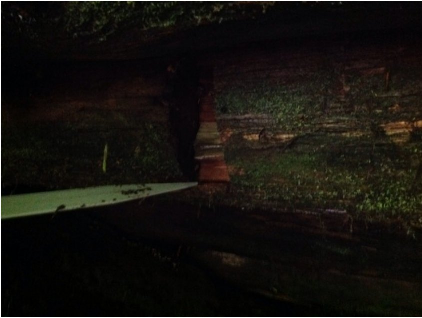
Stringer10 missing wood
