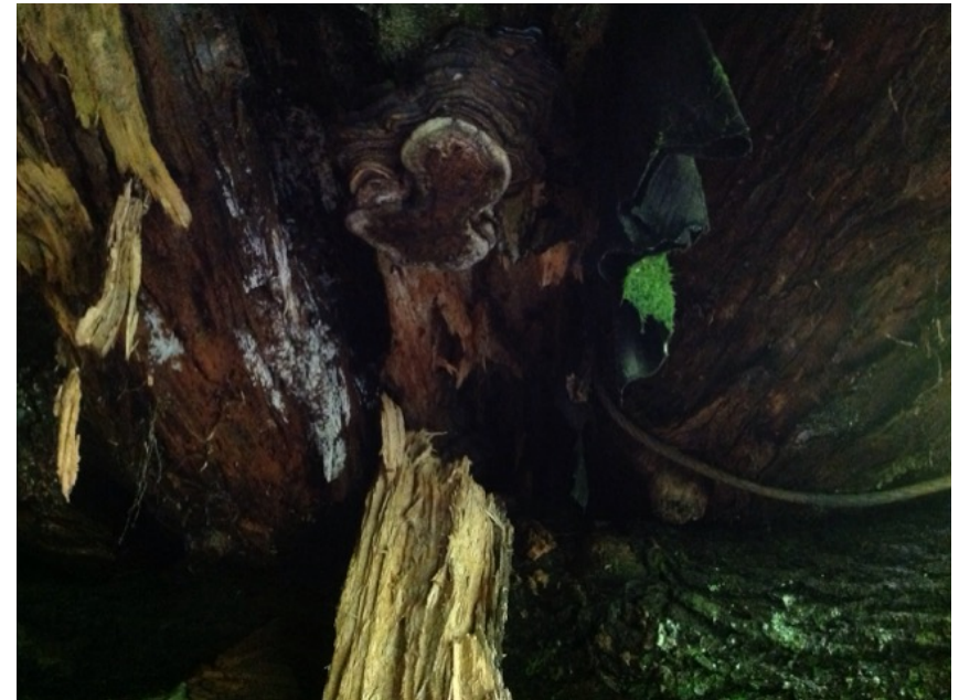
stringer 13 conk and rot
