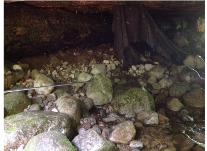
Left Bank Abutment when facing downstream
