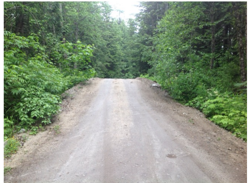
Approach from Left Bank when facing downstream
